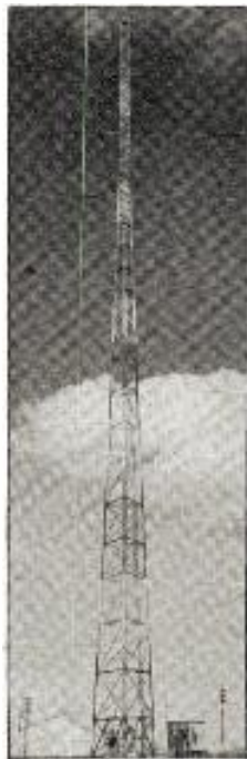
KAA-284, Owatonna, Minn., Northern Natural Gas Co. Truscon Self-Supporting Tower, 260 feet high.
