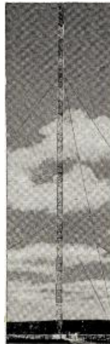
WHDH, Boston, Mass. Three Truscon Guyed Towers; 565 feet, 606 feet, and 645 feet high.
