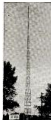
WTCB, Shawano, Wisconsin. Truscon Self-Supporting Tower, 240 feet high.
